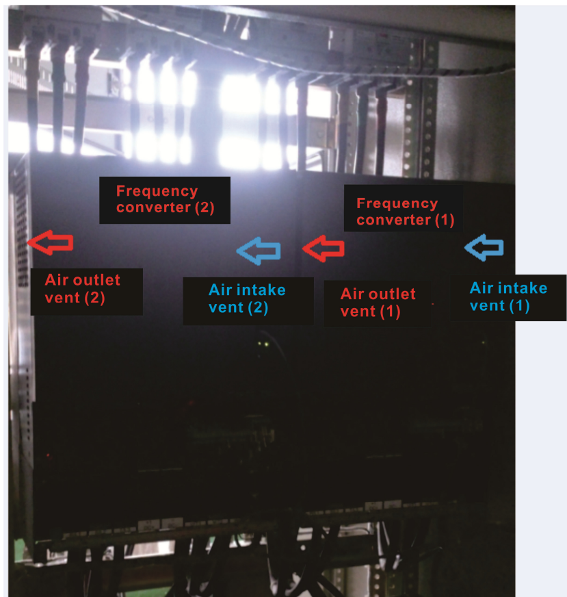
Improper Installation
