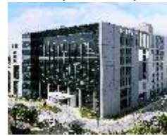
Taoyuan Technology Center (Green Building)
